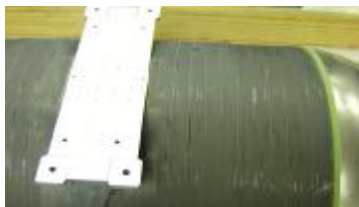
Figure 2: A Bonded Bracket
